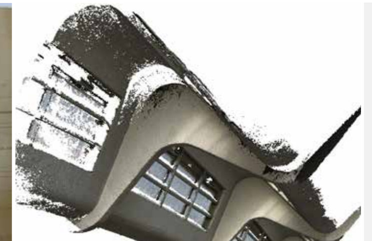
3c 5.9. (left): An in-depth study of the wave element of the Hall B vault in a very detailed drawing by Pier Luigi Nervi (CSAC, Università di Parma, courtesy Fondation PLN Project); (right) a view of the point cloud derived from close range photogrammetry of the same constructive element.
