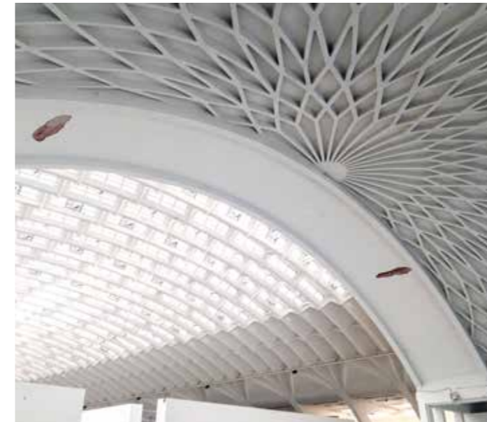
3b 1.1 (above): The wave vault of Hall B and the so-called SAP vault (reinforced concrete-brick vault) with some decay have been investigated in depth. (below) A diagram of the studied curves (dashed blue line for SAP vault and dashed red line for waved vault) overlapped to the transversal section of Hall B.
