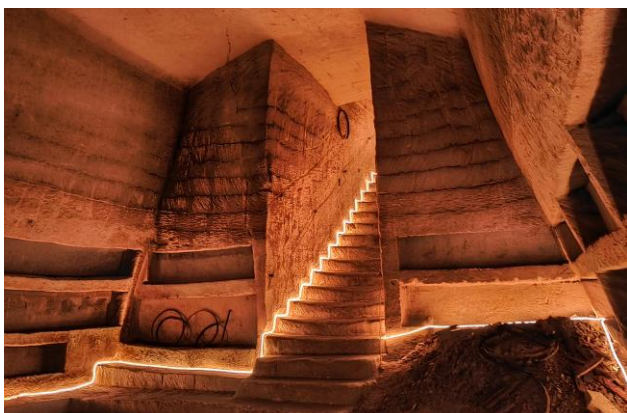
Figure 2. Image within the 'Cantina del Principe' artificial cave, research case study, revealing remnants of block excavation on the walls.
