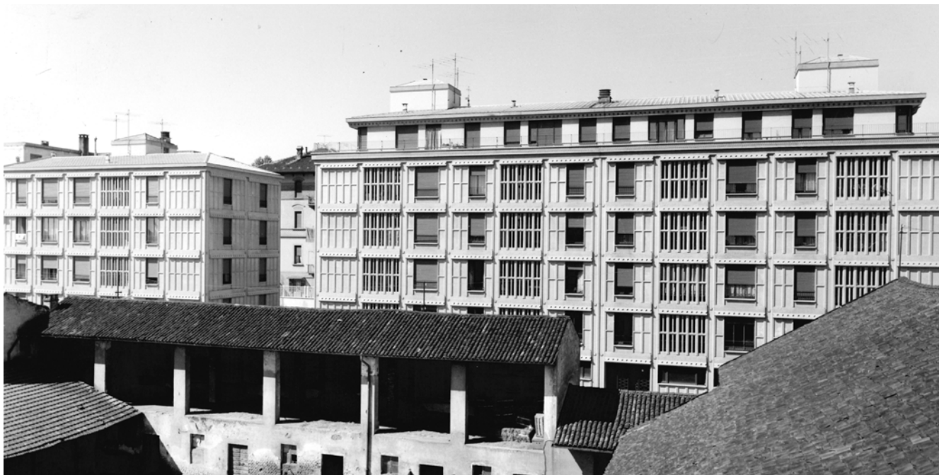
Figure 1. The VFG buildings, Novara, 1957–60. (CASVA, AA Archive collection, photo by Dino Sala).
