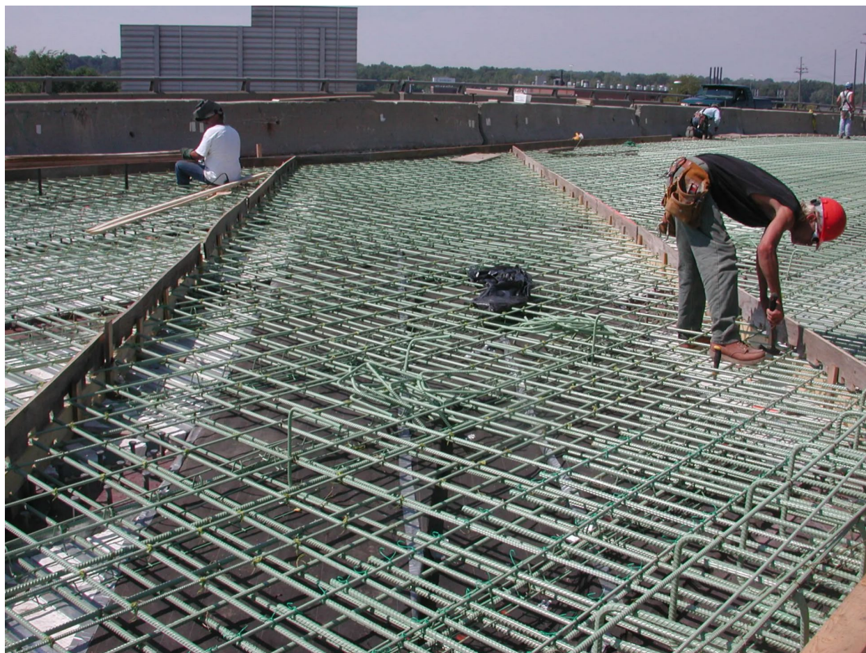
Fig. 4 Traditional construction site: The placing of reinforcements
