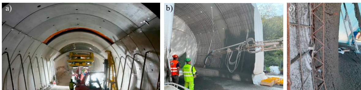
Fig. 7 a) “Colle Marino” tunnel construction site – relining by high strength shotcrete b) and c) “San Fermo” tunnel - Field test of shotcrete application
