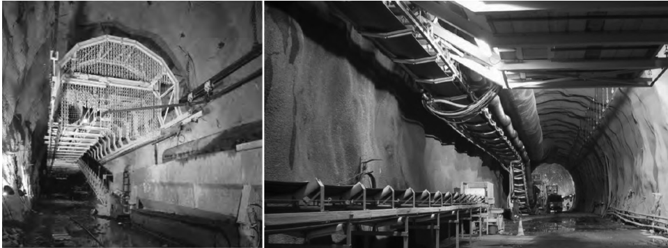
Figure 6.17 View of equipment from tunnel face; crusher and hanged conveyer belt.
