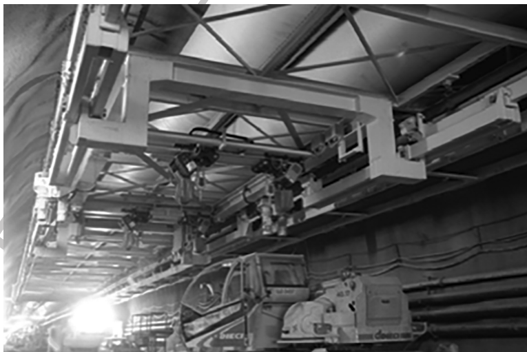
Figure 6.20 The 15 t heavy-duty crane in the invert construction area. The 66 m long invert platform may be moved accordingly to the heading platform.
