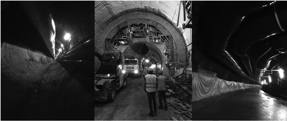
Figure 6.54 Ducts installation inside tunnel.
