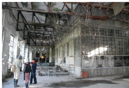
Figure 8. The Annual Art Festival held at Hokutan Thermal Power Plant. Source: https://www.shimizusawa.com/hatsuden (accessed on 6 April 2020).
