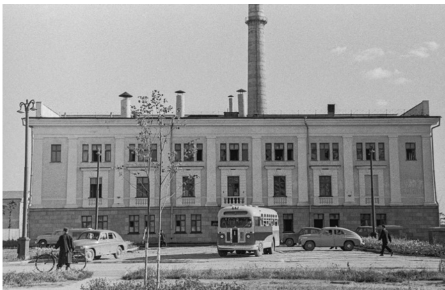
Figure 9.2 Obninsk Power Station, 1954
