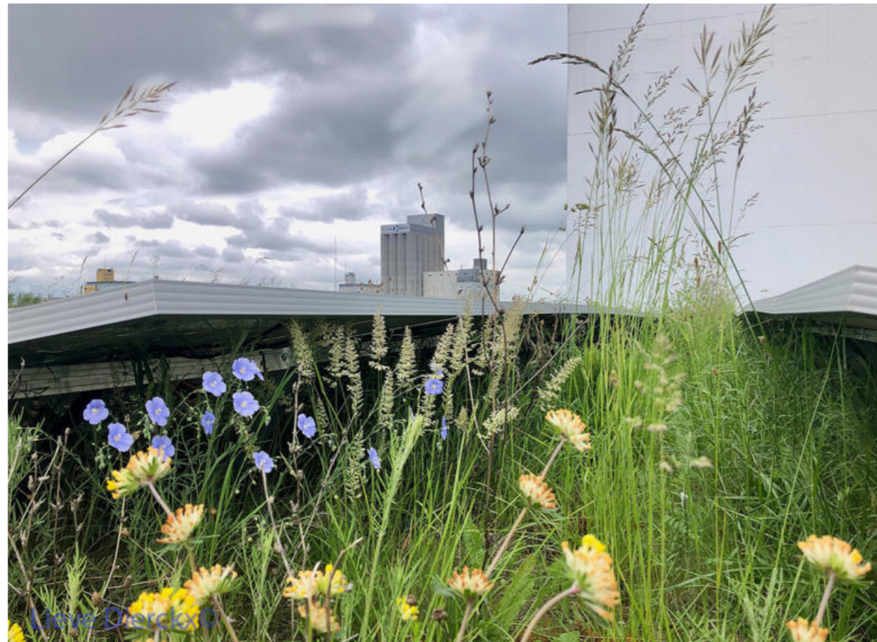
Figure 1: Roof of the shopping centre Stücki, Basel, Switzerland. Plant species rich extensive green roof with photovoltaic installation. Copyright: L. Dierckx
