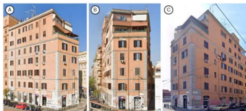
Fig. 2. Building facades prior to thermal insulation interventions: south-east (A), north-east (B), north-west (C). From [15].
