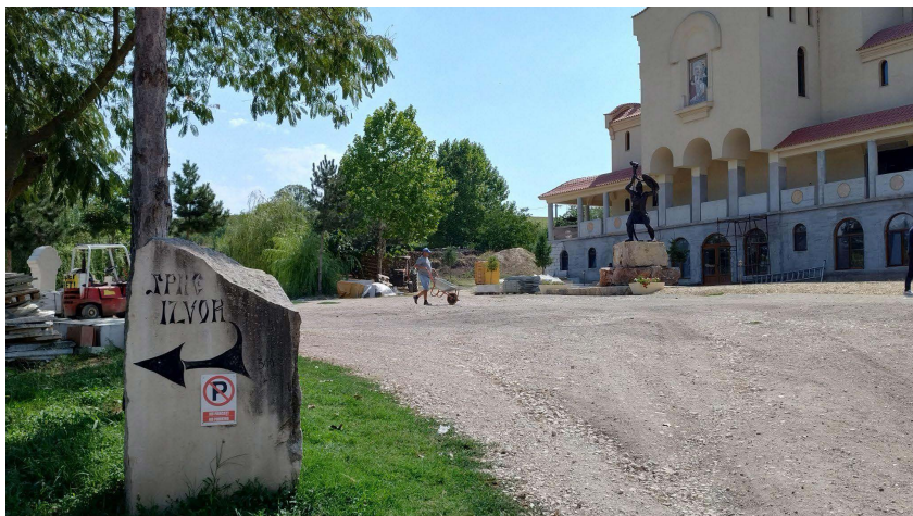
Figure 12: At the construction site of the new church. The stone indicates the way to the spring. Photograph by Giuseppe Tateo.
