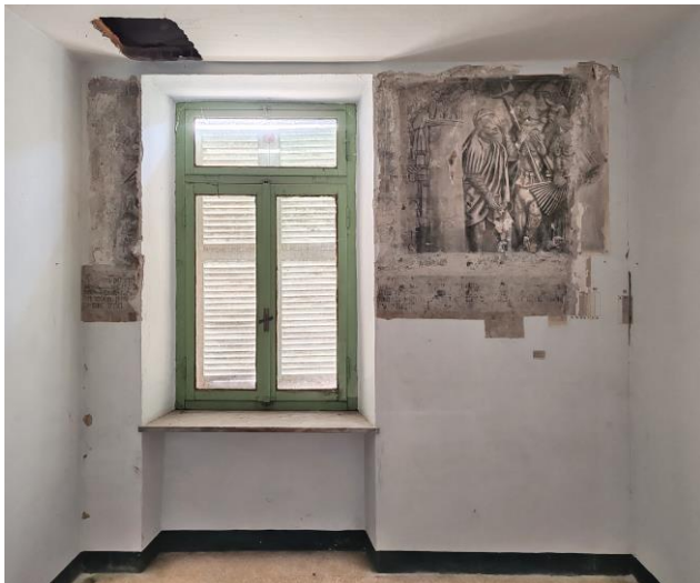
Fig. 3: One of the frescoed rooms on the second floor of the north wing belonging to an originally unified hall that was, over time, split with partitions and lowered with suspended ceilings. Note the superficial holes from the recent stratigraphic surveys and restoration of the building, as well as the deeper one to investigate its upward development (R. Rudiero 2024)
