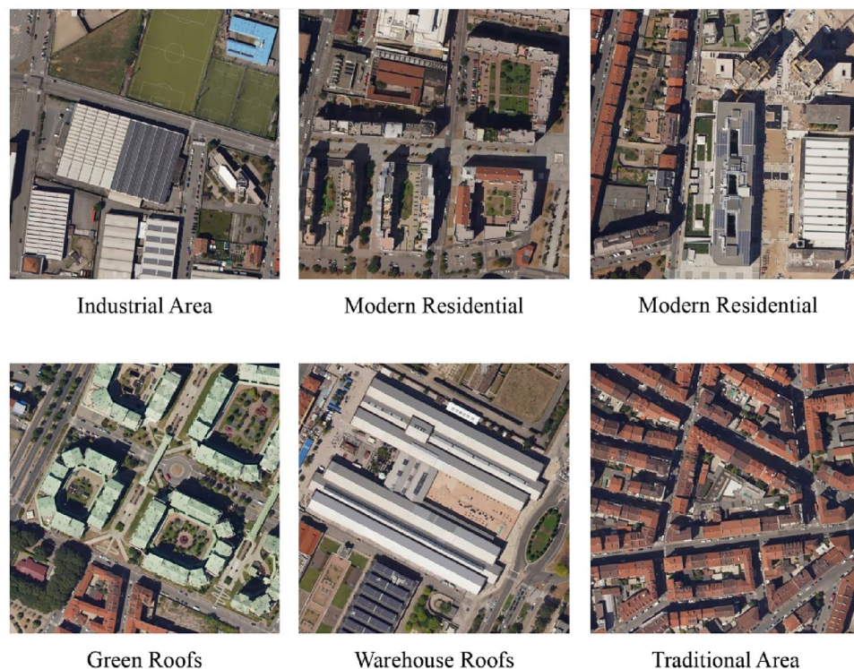
Figure 1. Example of different roof types in the case study.
