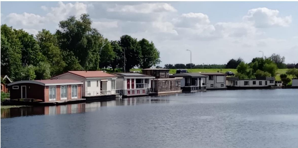
Figure 57: floating houses outside Gorinchem (my photo).
