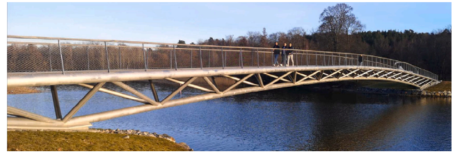
Fig. 1. The Folke Bernadotte Bridge in Djurgården, Stockholm, Sweden.
