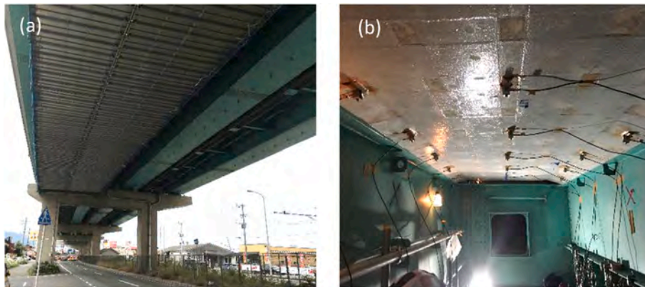
Fig. 13. (a) Tested highway bridge, (b) sensor arrangement for the measurement before repair.
