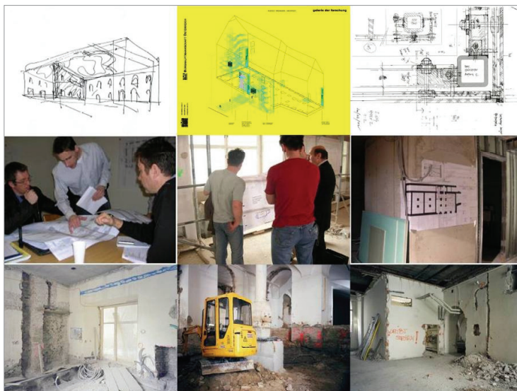
Figure 1. Renovation in the making. (Photos and collage: the author)
