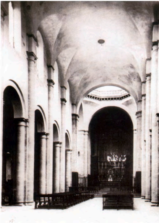
Fig. 2. Period picture, showing the same shot as in the previous picture, representing the condition of the cathedral after the works (1926–1928). The first, glaring evidence is the removal of chains at the arches of the vault in the nave.
