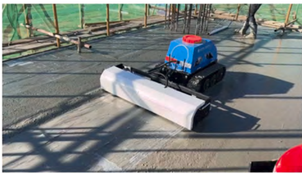
Fig. 15. Robot plastic film curing operation.
