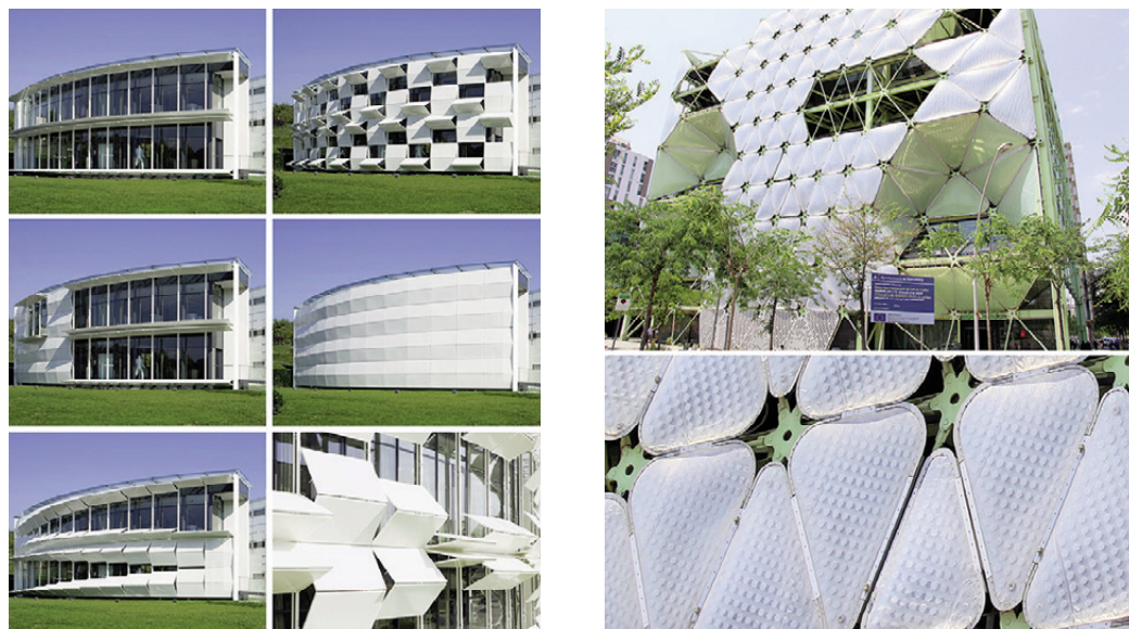
Fig. 4 | Kiefer Technic Showroom (2006-07) in Graz, designed by Ernst Giselbrecht and Partner ZT GmbH (source: archtonic.com; credit: P. Ott, 2010).
