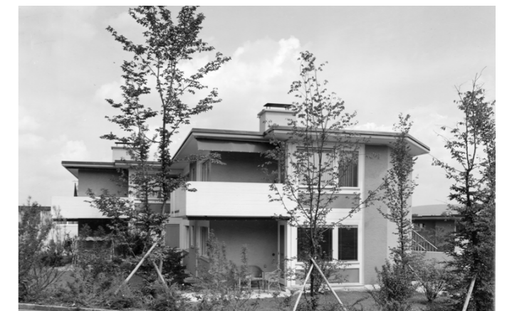
Rebenstrasse 74/76, two-family freestanding house in individual ownership, Zurich, District Leimbach, 1964 (© photo: Wolf-Bender's Erben, Baugeschichtliches Archiv/City of Zurich, 1965)
