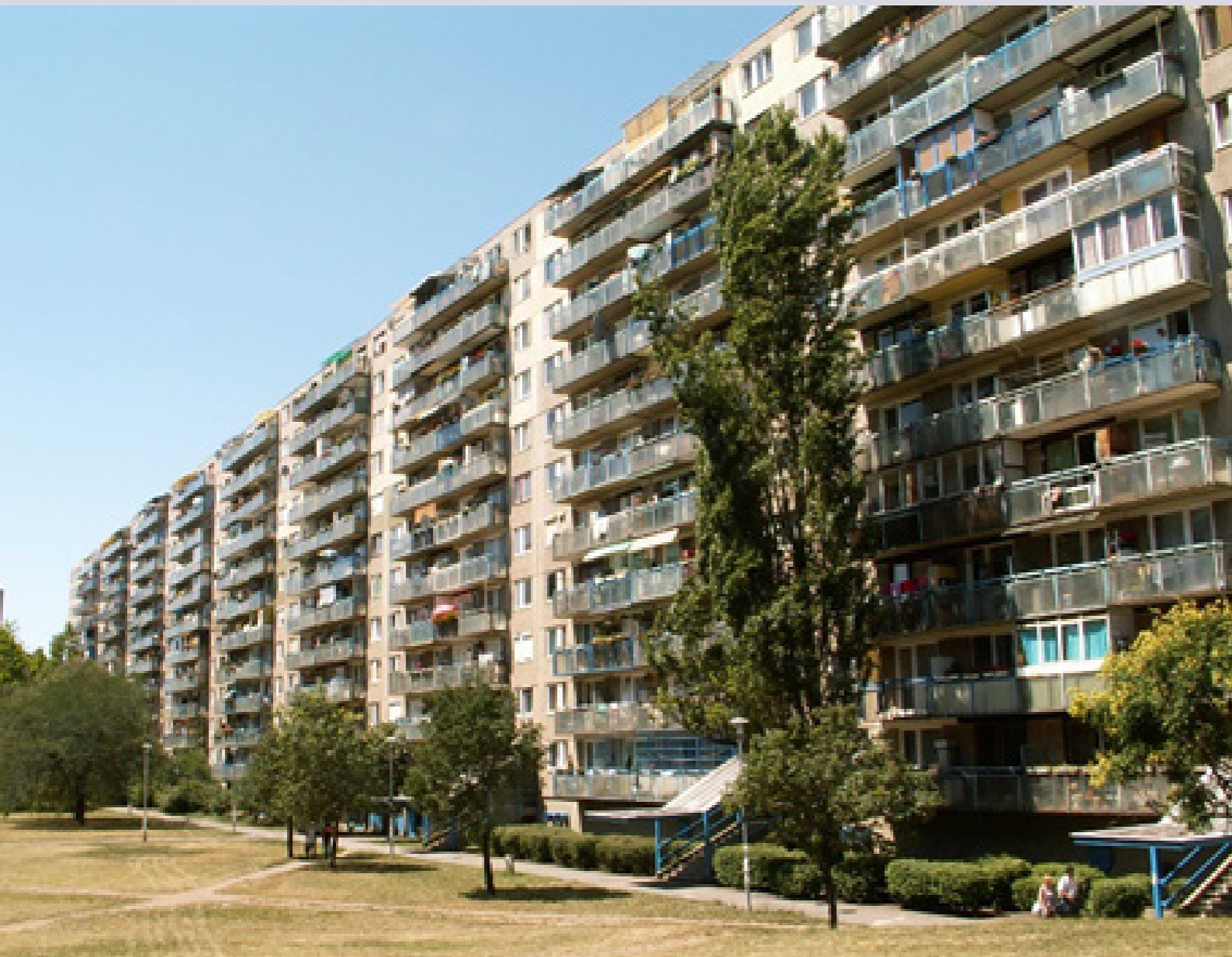
Havana housing estate built by prefab technology in the 18th district of Budapest in the second half of the 1970s (© photo: Tamás Egedy, 2017)
