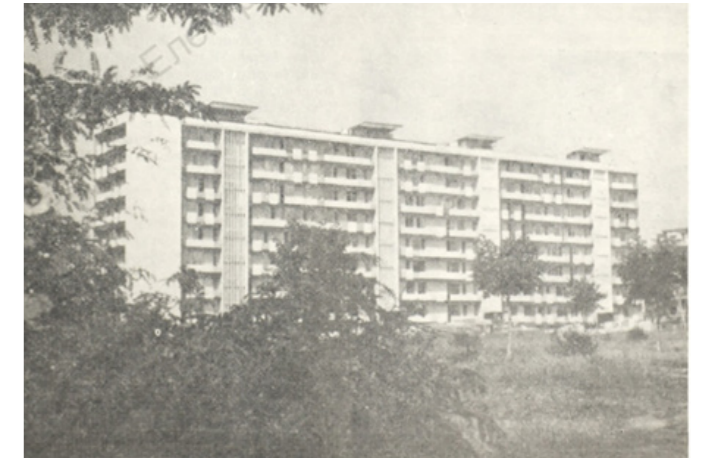
Residential building (block) in Sofia, Hipodroma residential estate, built ca. 1960; source: Stoychev [1976].
