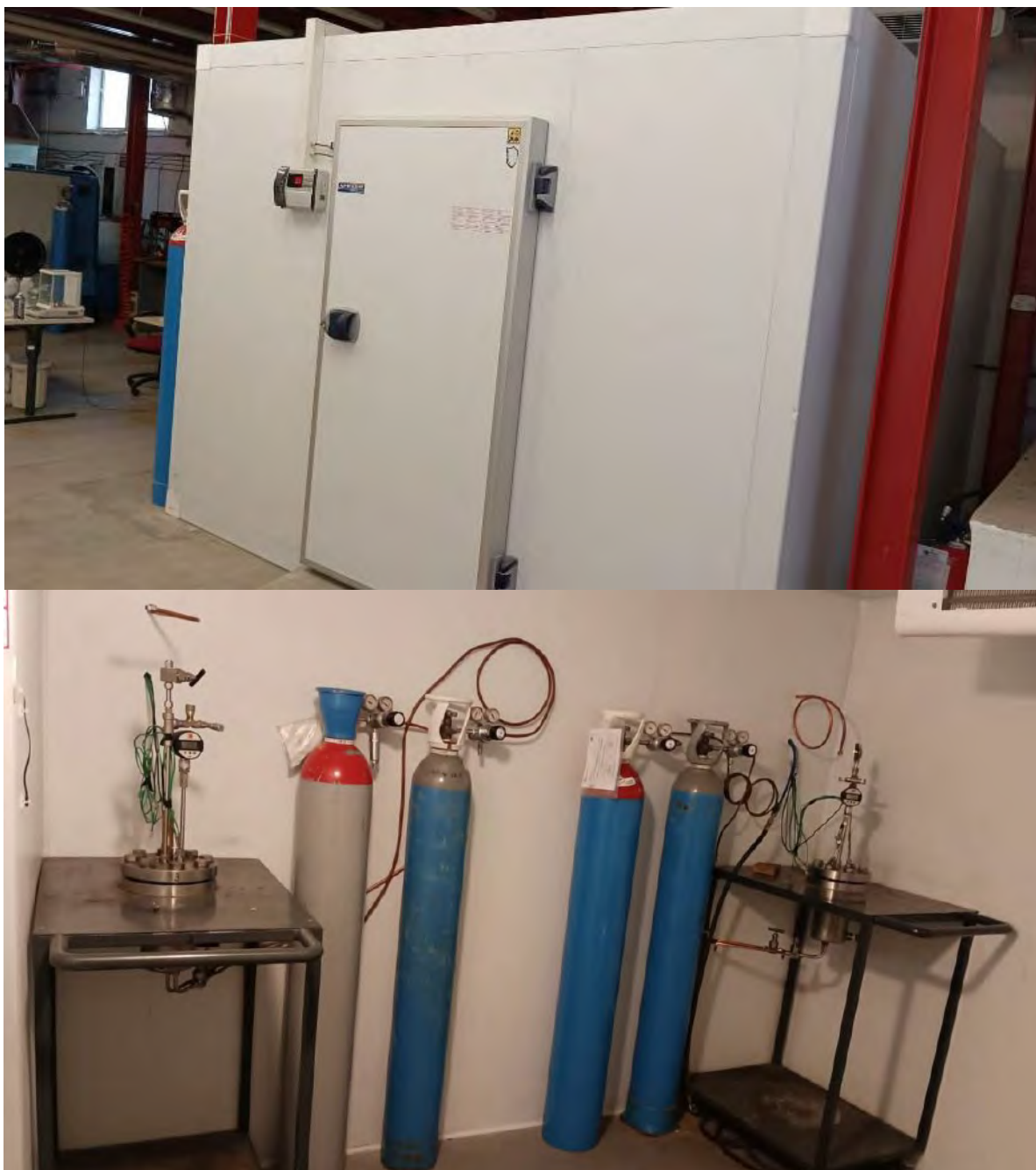
Figure 5. The new reactors in the refrigerated room.
