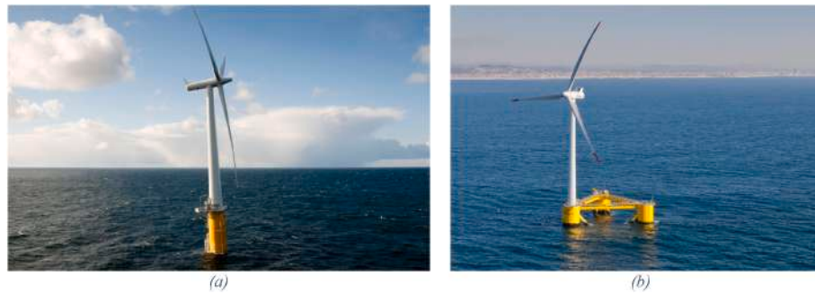
Fig. 4. Hywind (a) and WindFloat (b) floating offshore wind turbines [63,64].
