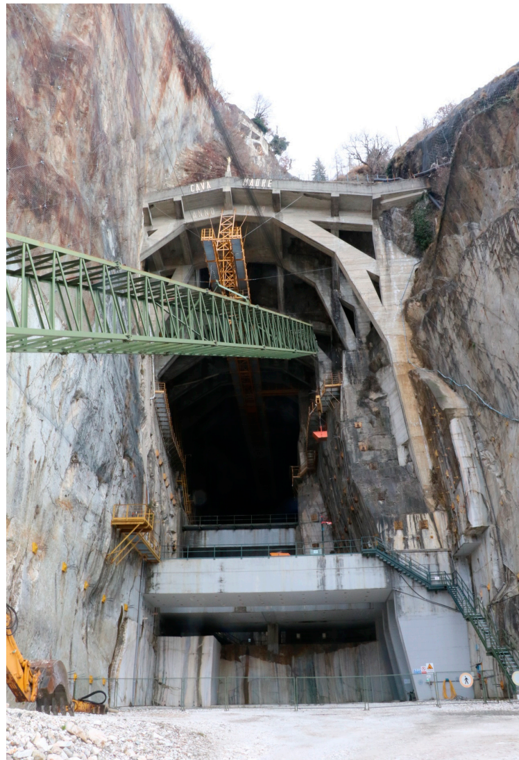
Figure 1. View of the entrance area of the Cava Madre di Candoglia after the lateral expansion works of the cavern and the reconstruction of the contrasting structures on the side walls.
