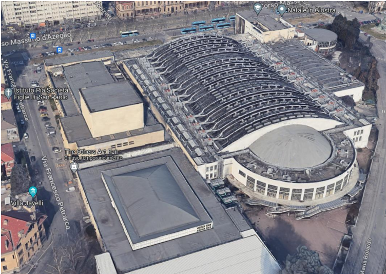
Fig. 1. View of the Hall B structure ( https://www.google.it/maps/@45.0467459,7.6839451,144a,35y,318.98h,56.88t/data=!3m1!1e3 ).
