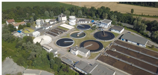
Fig. 1. Aerial view of the wastewater treatment plant located in Collegno (Italy) and managed by SMAT S.p.a.
