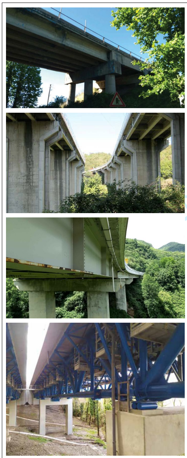
Figure 1 Some cases of bridges assessed by ASPI with the external review by Politecnico di Torino.
