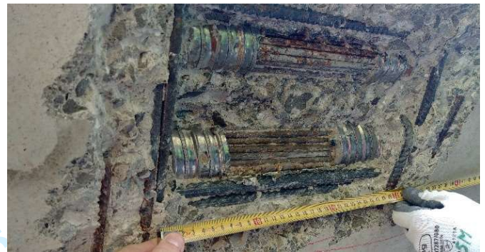
Figure 5 Removal of concrete cover to assess tendon layout and relevant deterioration.
