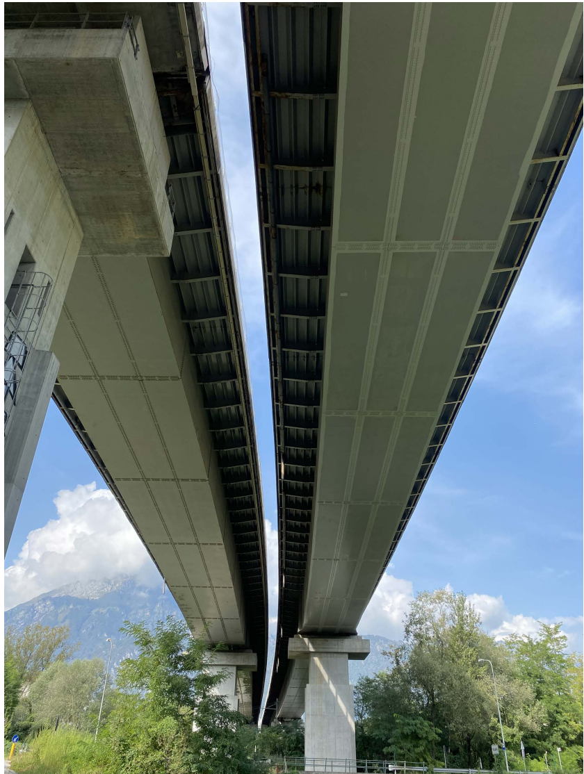
Figure 2. View of the intrados of the central span.
