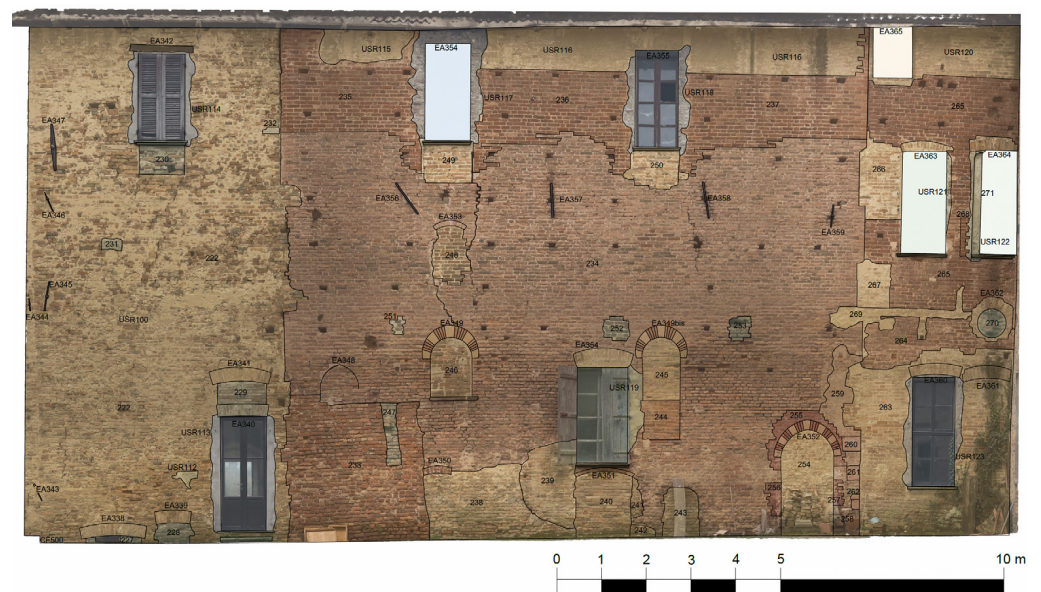
Figure 14. Part of the south front of the internal courtyard: stratigraphic units (USM, USR, and EA), analysis, and interpretation.
