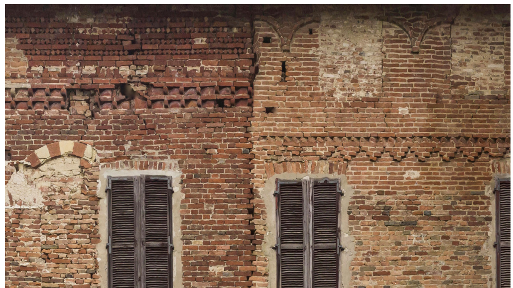
Figure 12. Section of the central part of the west front of the castle: on the left side, the earlier masonry and decorations (Period I), while on the right side, the connected masonry and Ghibelline decorations related to Period III.
