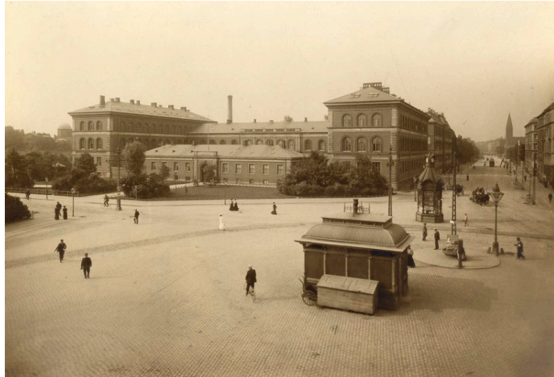
Fig. 1. The Polytechnic School, Copenhagen, ca. 1904–06. [courtesy of Danmarks Tekniske Højskoles Billedsamling/DTU Photographic Archives].
