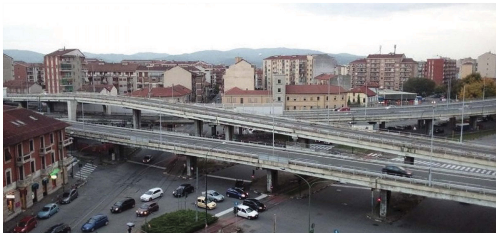
Figure 1. An historical view of the Corso Grosseto viaduct.
