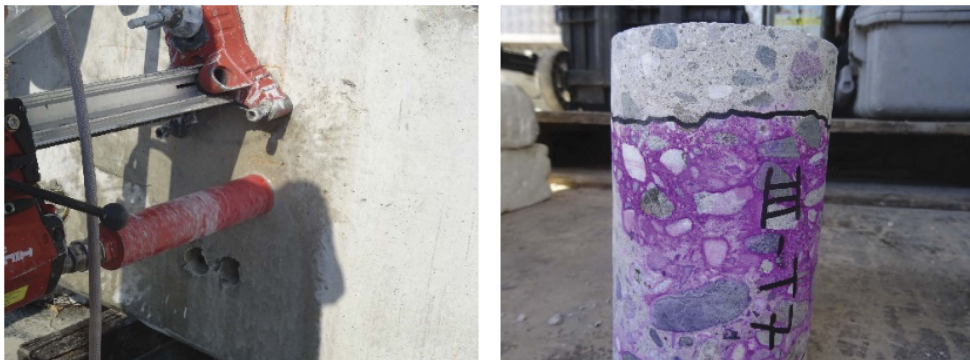
Figure 4. Coring of samples from PC bridge deck beams.
