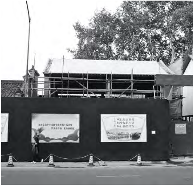
Fig. 03 - Urban regeneration works in XiaoXiHu block
