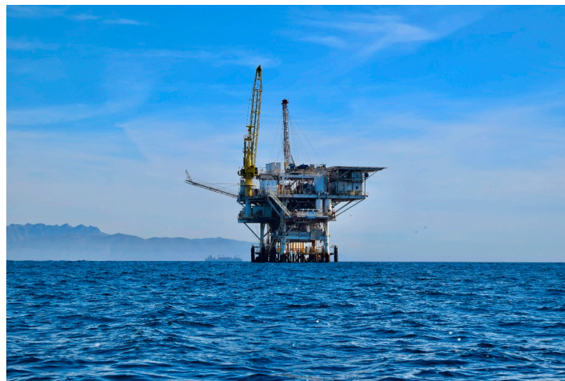
Figure 1. Typical oil and gas offshore platform [Photo by Zachary Theodore on Unsplash [18]].
