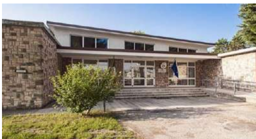
Fig. 1 – Real image of the school building under study
