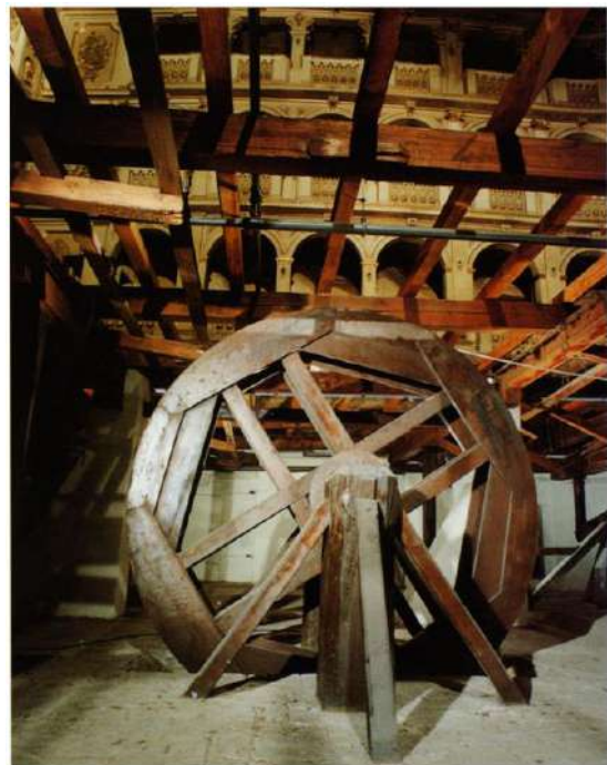
Fig. 4 – Wooden mechanical system located beneath the finish floor of the stalls
