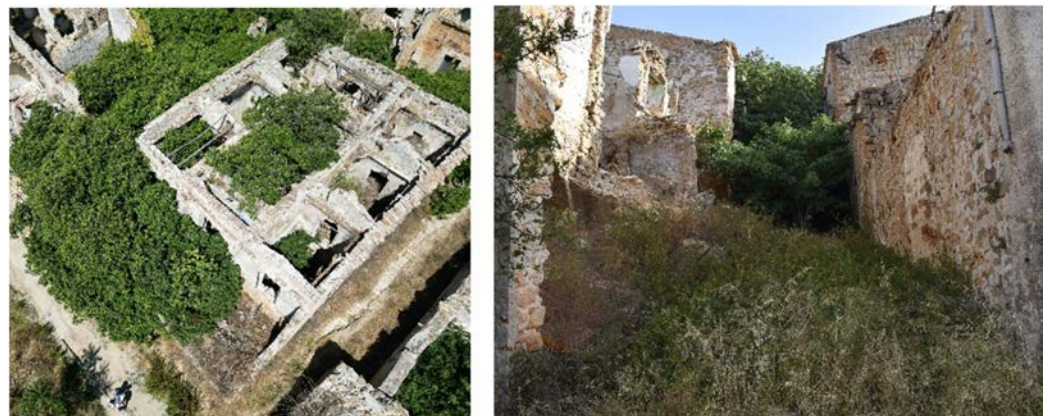
Figure 9. Presence of trees and weedy ground vegetation compromising, in some cases, masonry structures themselves (authors’ photos).
