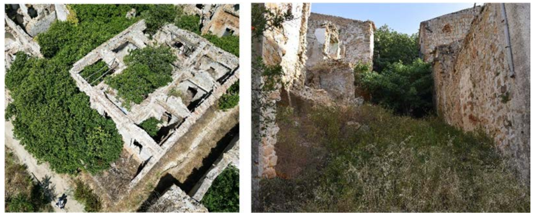
Figure 9. Presence of trees and weedy ground vegetation compromising, in some cases, masonry structures themselves (authors’ photos).
