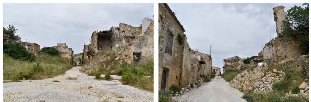
Figure 5. Views of Corso Umberto I from the Piazza Elimo and of an upper parallel road (authors' photos).
