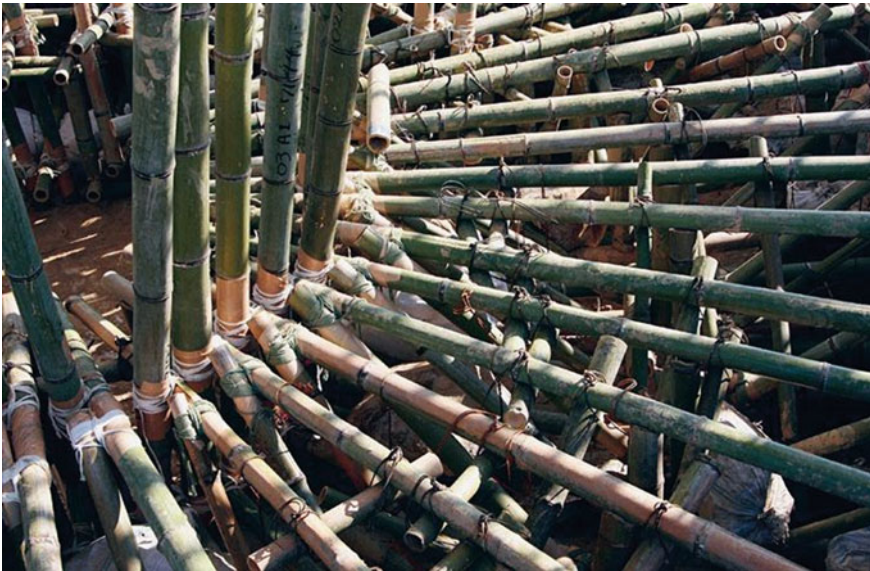
Fig. 33.4 Structure of the Bamboo Ark consists of radially arranged frames, composed of a base truss and arches. The culms were harvested from a nearby grove. Photo Toki Hirokazu
