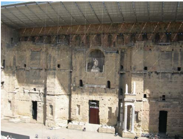
Fig. 1 – The stage front of the theatre in Orange with the new roof to contain all the installations necessary for cultural performances
