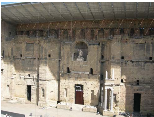
Fig. 1 – The stage front of the theatre in Orange with the new roof to contain all the installations necessary for cultural performances
