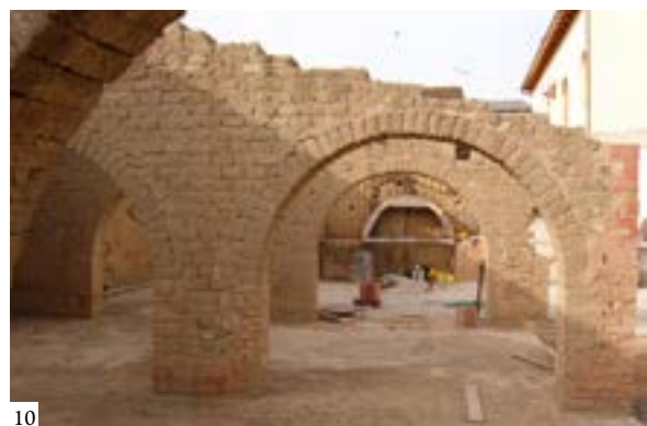
Figure 7: In the reconstruction work of building B, the reuse of original ladiri in good condition was frequent. The earth derived from the demolition, heterogeneous and with spurious materials, was not reused within the construction site, but was instead reused to fill the land where the earth used for the new bricks was extracted from. (Ignazio Garau)
