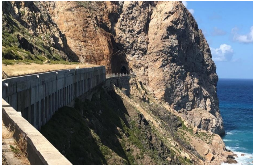
Fig. 1. Capo Calavà site, where part of the artificial rockfall sheltering tunnel is also visible.
