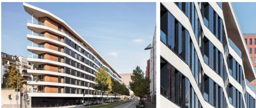
Fig. 29.11 Newly built apartment building Aktiv-Stadthaus
