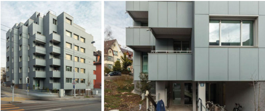
Fig. 29.12 Renovation of an apartment building
