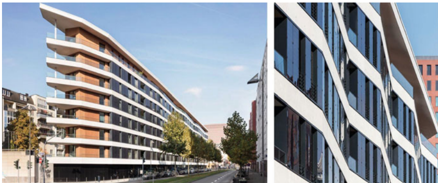
Fig. 29.11 Newly built apartment building Aktiv-Stadthaus
