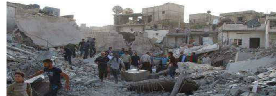
Fig.8. Destroyed concrete buildings in Aleppo, Syria (Aljazeera, 2016).
