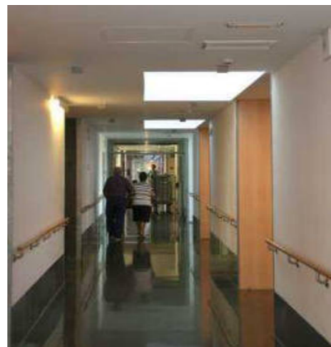
Fig.8. In-patient ward corridor. Hospital de Dénia.
