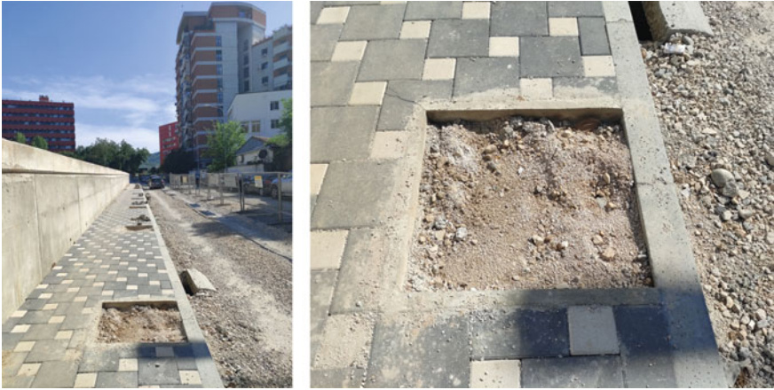
Fig. 11.3 Project for new Green infrastructure added to the renewal of the road surface and pedestrian pavement in Rruga Dora D'Istria in Tirana, Albania. The width of the pavement is 2 m, while the distance between the two tree boxes is around 5 m. Source the author
