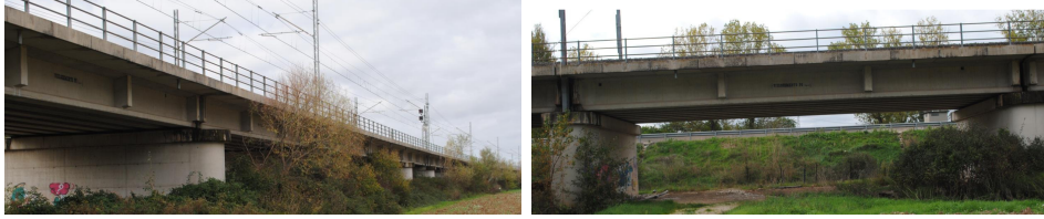
Figure 10: Views of the viaduct and of a sample span.
