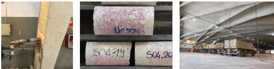
Fig. 17. Pavilion V: Extraction of concrete sample from a strut-beam (left); carbonation tests on sample of the ribs (centre); view of the static tests with trucks connected to the ribs through jacks (right).
