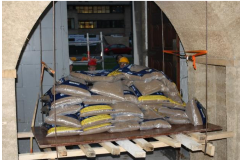
Figure 3: Structural testing of the hemp lime vault
