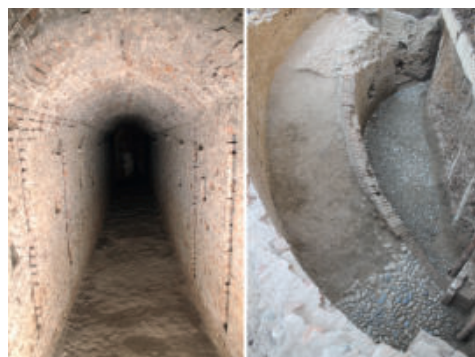
Fig. 3- Communication gallery between the ravelin and the citadel and access ramp to the rampart of the ravelin under excavation (photos by GEA S.A.R.T. s.a.s.)
