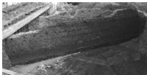
Fig. 2- The eastern side of the gorge front of the Rivellino degli Invalidi. In the foreground, a section of the citadel's main moat (photo by GEA S.A.R.T. s.a.s., Micheletto et al, 2020)
