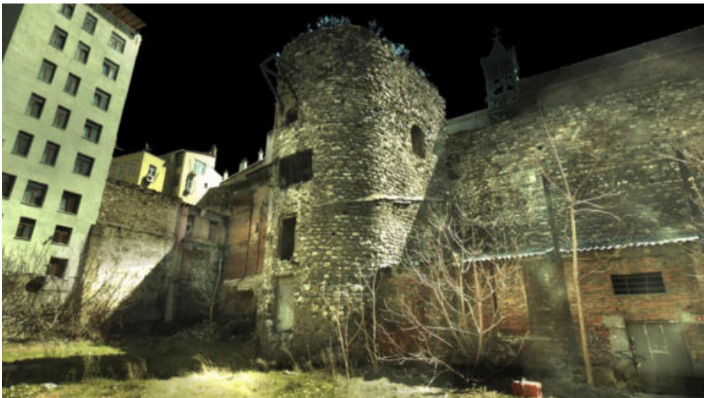
Fig. 5- View of Tower one from the point cloud, colored map mode, panoramic view
