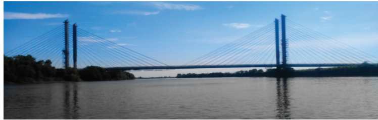
Figure 2. The Rio Papaloapan Bridge.
